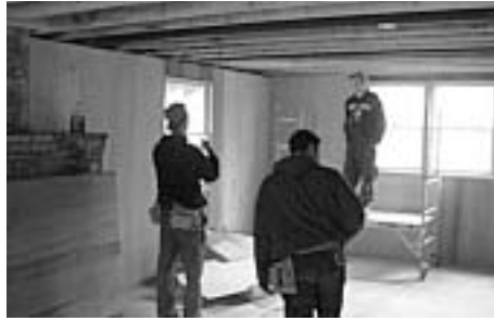
New walls and floor are in, ceiling is almost finished.
