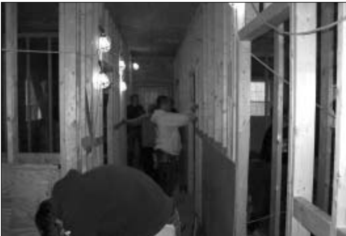
General Nash Chapter comes through again. Drywall and wiring started.
