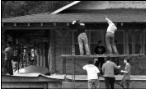
Staining work is begun on Unami Lodge
